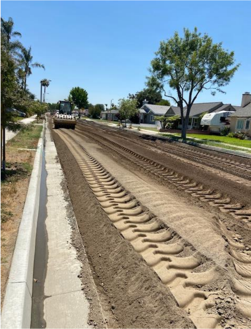
Cement Stabilized Pulverized Base Operation
