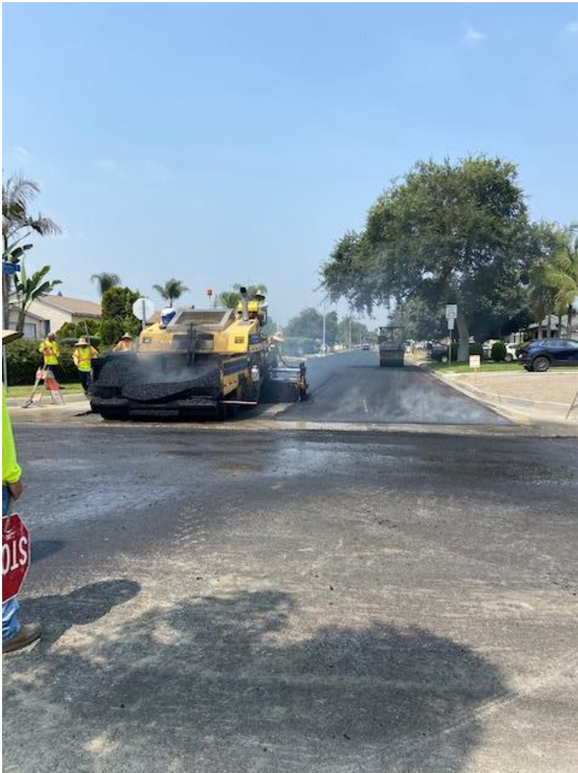
Asphalt Rubber Hot Mix
