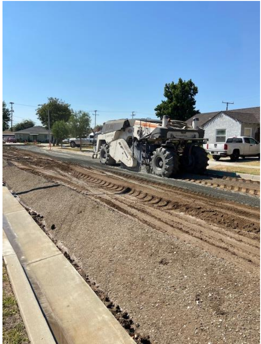
Cement Stabilized Pulverized Base Operation
